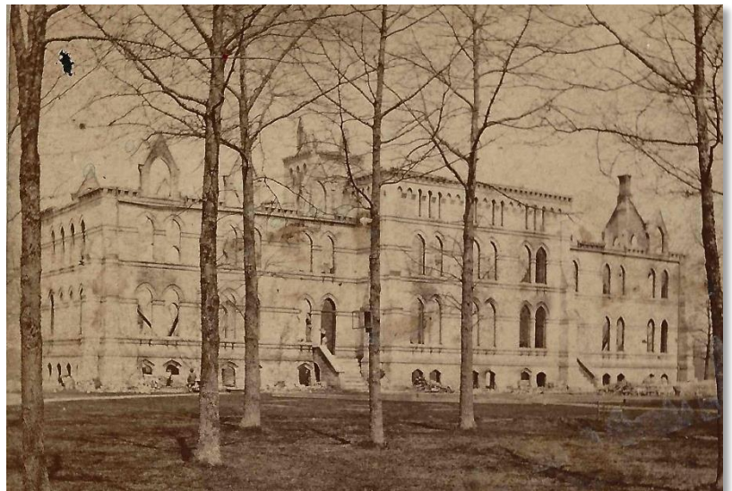
Figure 3 Taylor Hall After the Fire (1875)
